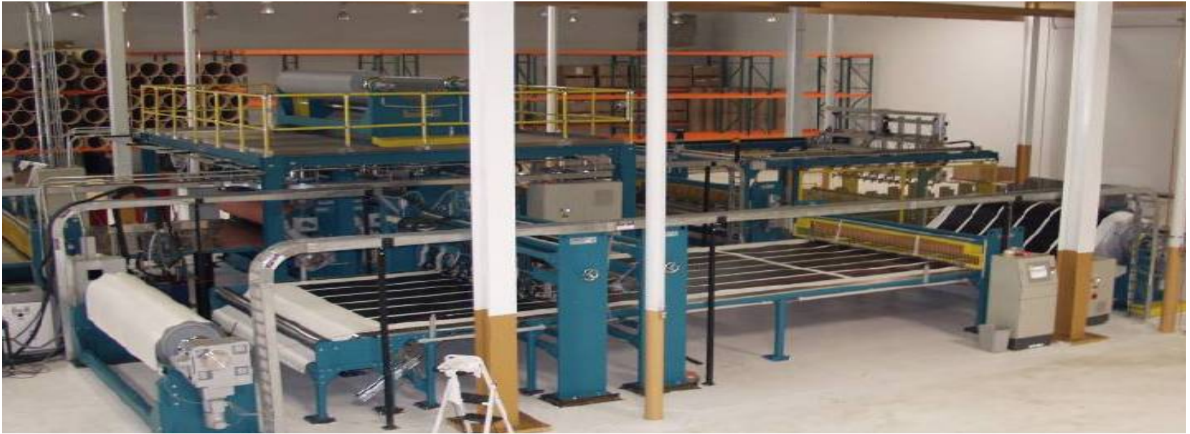
Production facility in Los Angeles
